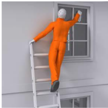
Figure 3 Incorrect – overreaching and not maintaining three points of contact
